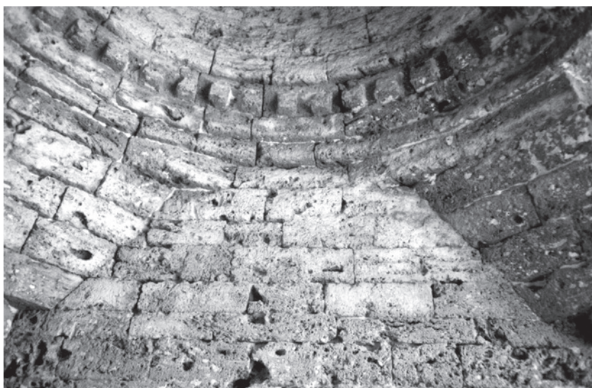
Fig. 33. Kāfirkoṭ, Temple A, squinches as transition from sanctum to dome.
