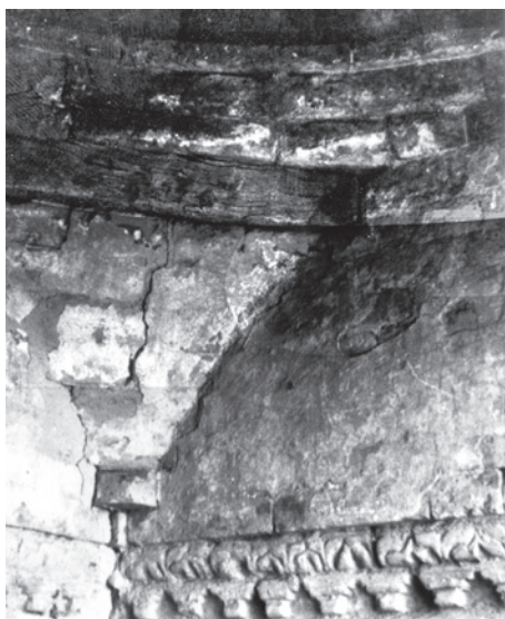
Fig. 38. Kālar, brick temple, squinch with wooden beam above.
