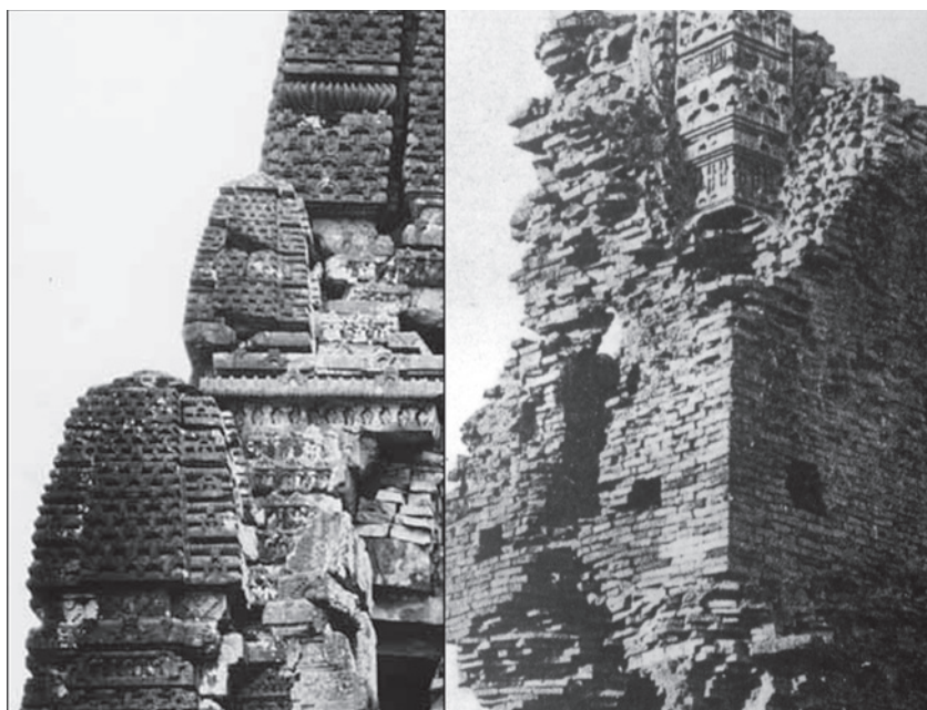
Fig. 121. Pattan Munāra, brick temple (right), detail of damaged tower before conservation; Gyaraspur, Madhya Pradesh, Mālādevī Temple, ca. 950 (left), detail of multi-spired tower.
