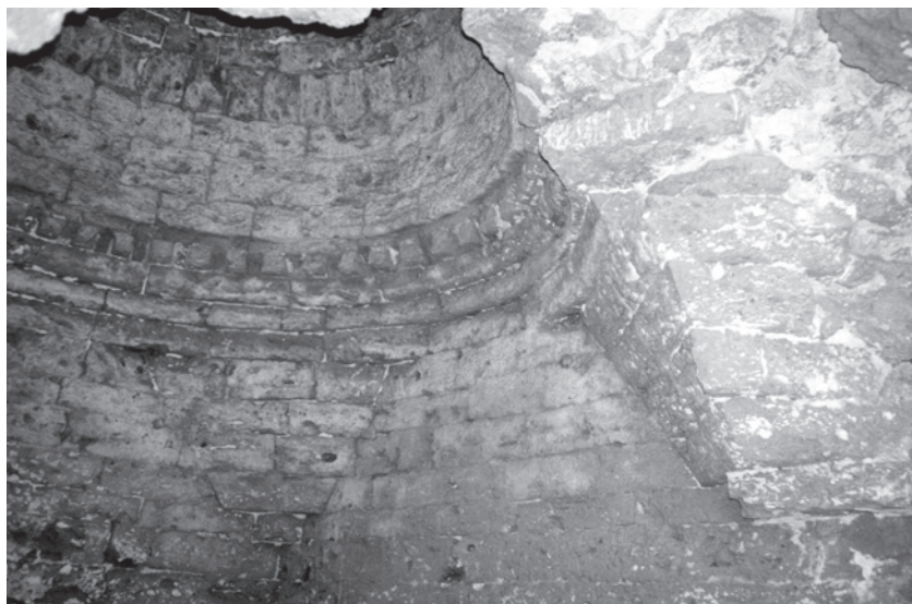
Fig. 34. Kāfirkoṭ, Temple A, squinches and dome.
