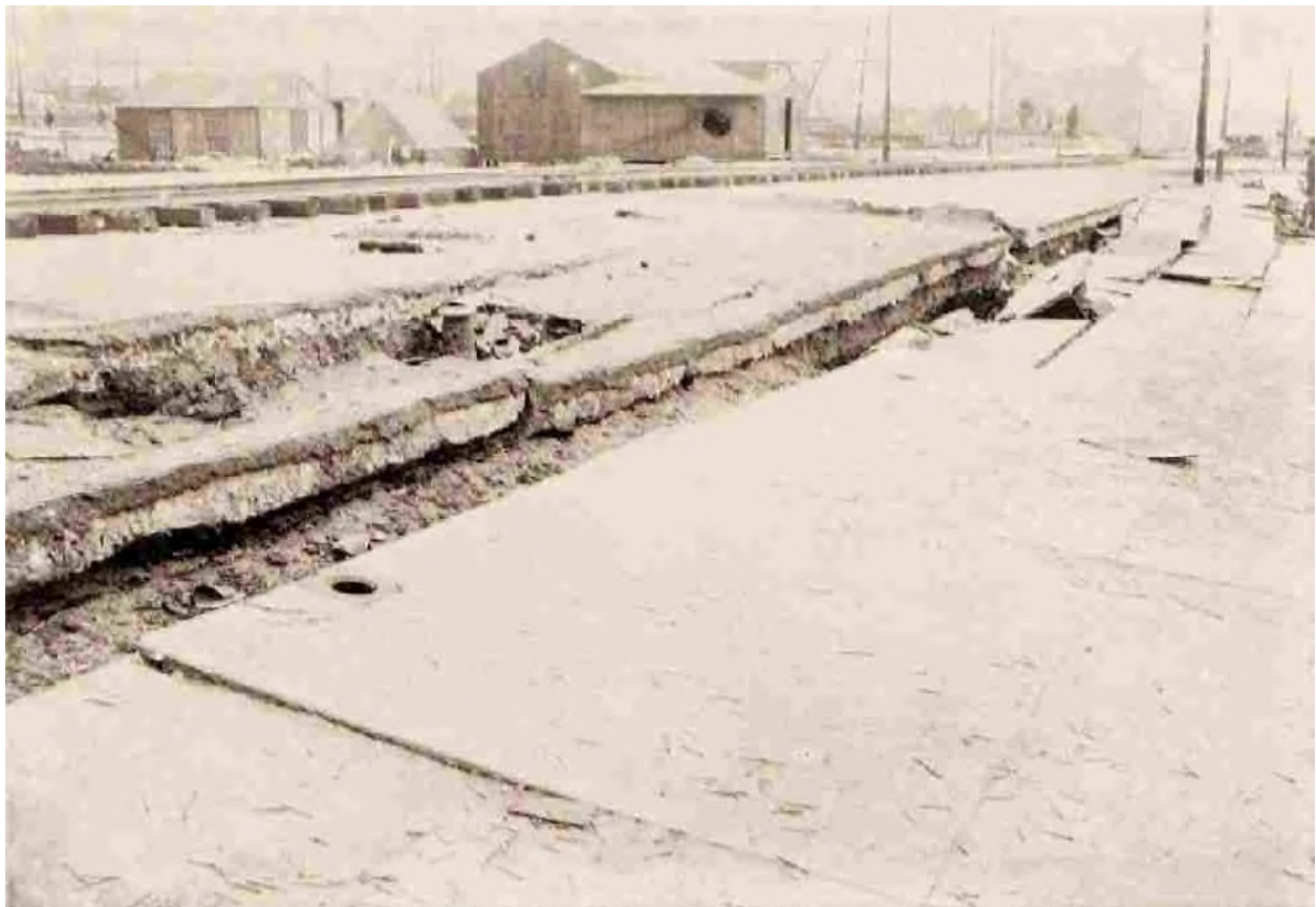
Effects of Shock: Separation of the Sidewalk from the Asphalt Paving on Capp Street, Between Seventeenth and Eighteenth Streets.
