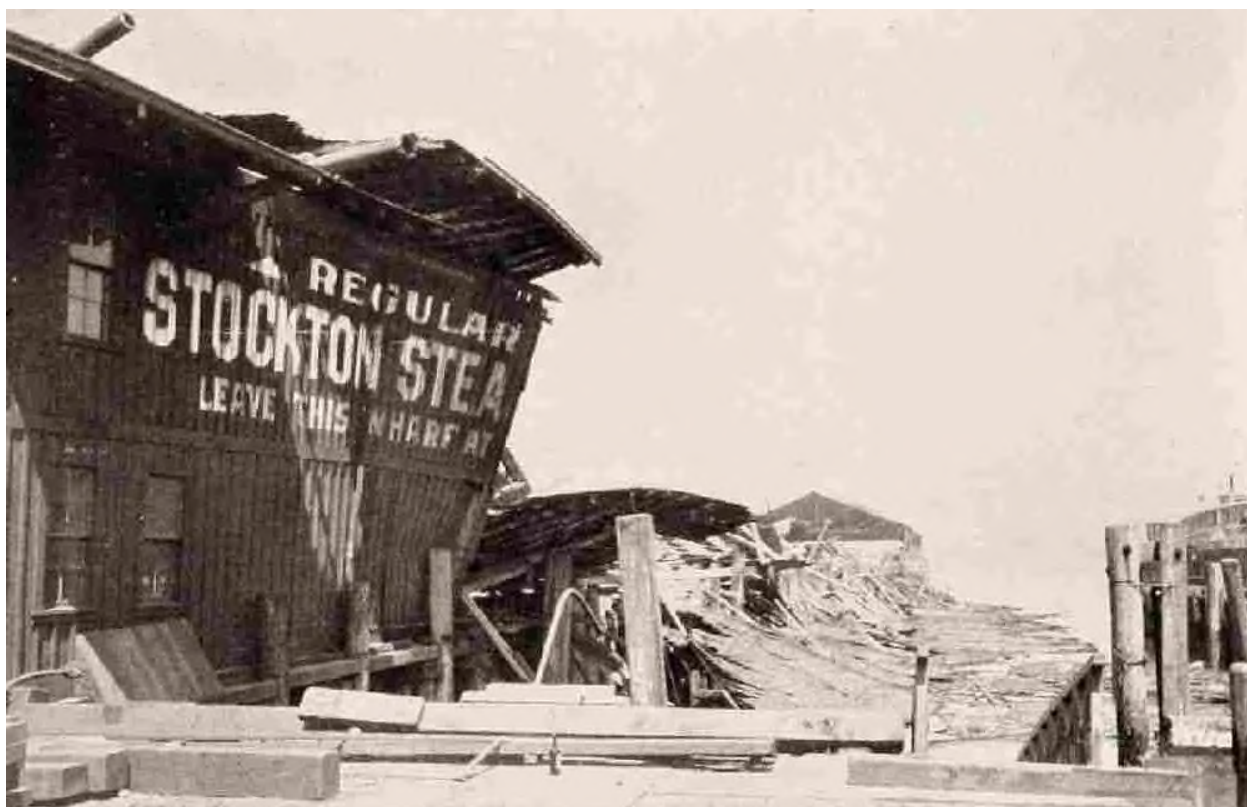
Effects of Shock: Collapse of the Stockton Steamer Wharf, Water Front, Near Ferry Building.
